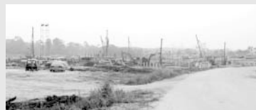
UCTS campus under construction (as at September 2012).
