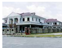
3. Stutong Avenue Link
