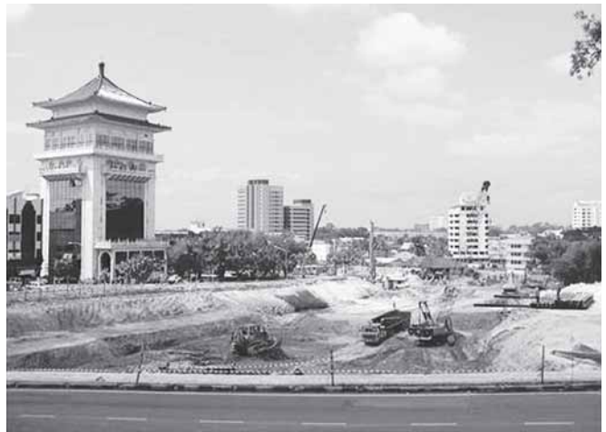
Novotel Under Construction in Kuching
