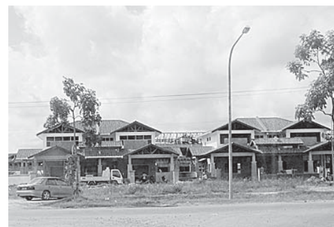
A new residential estate under construction at Jalan Stutong, Kuching
