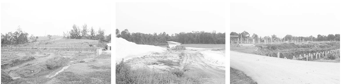
Various residential developments under construction in Bintulu
