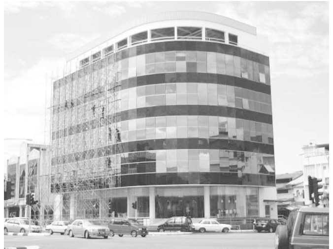
Workers adding in the finishing touch to TheLimeTree Hotel scheduled to open by end March 2009
