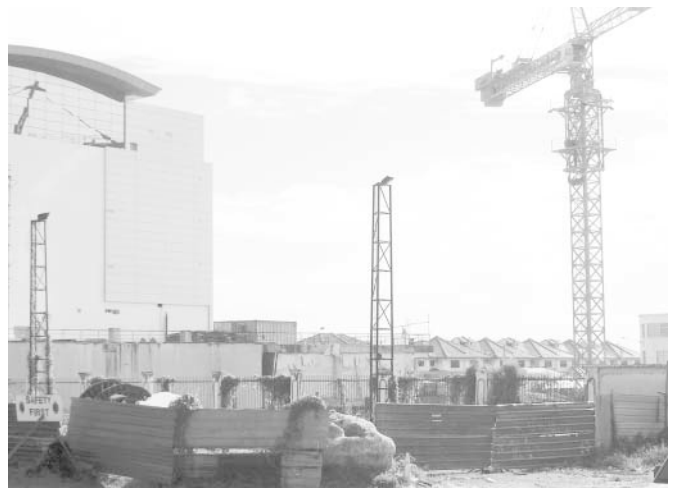
Boulevard Extension Site under construction
