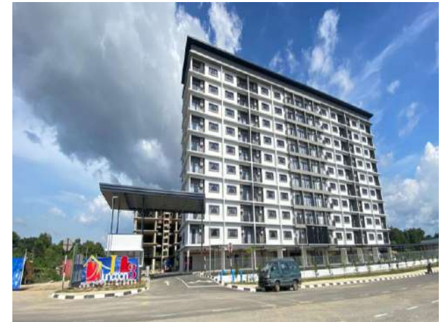
Junction 3 Apartment (Block 1), Bintulu
