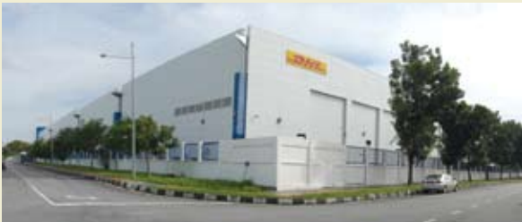
DHL warehouse-cum-office complex in Bayan Lepas Industrial Park
