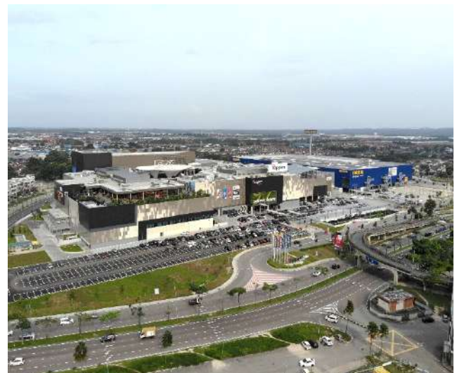
Toppen Shopping Centre Source: CBRE | WTW Research
