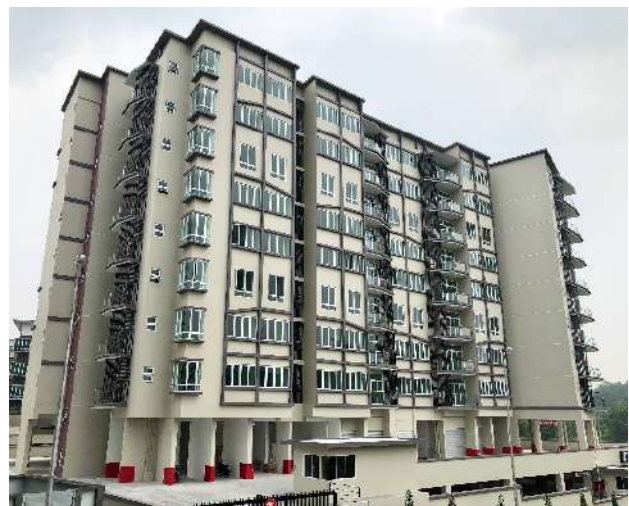
The Fifth Ryegates at Jalan Airport Source: WTWY Research
