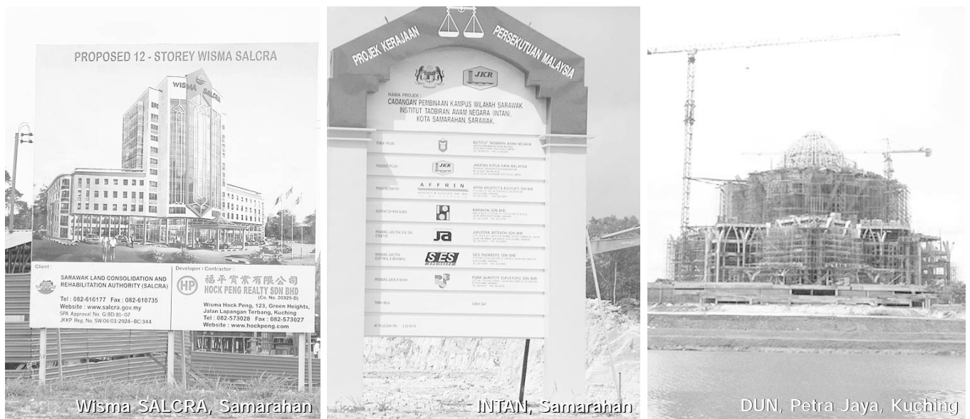
Some government institutions under construction
